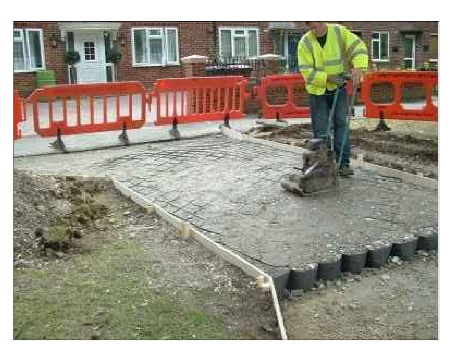
CELLULAR CONFINEMENT CONSTRUCTION TO PROTECT TREE ROOTS
